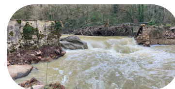
Dam failure following a flood (Bourgogne-Franche-Comté, France)
